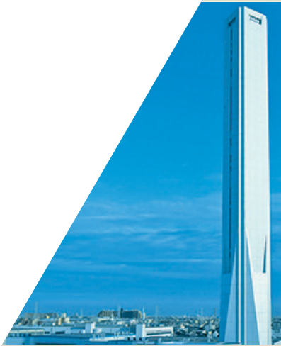
2007 Completed 173m tall elevator testing tower (world's tallest at the time)
