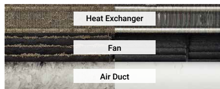
Simulated Comparison of Dirt on Heat Exchanger, Fan and Air Duct
