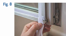
Join the ends of the tape to ensure a complete seal.
